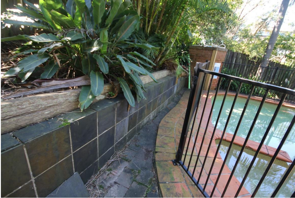
Plate 15: Existing slate covered Besser block retaining wall.
